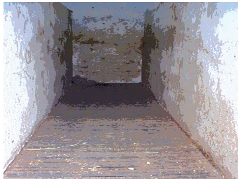
Fig. 8.5. Gratings over the plenum
