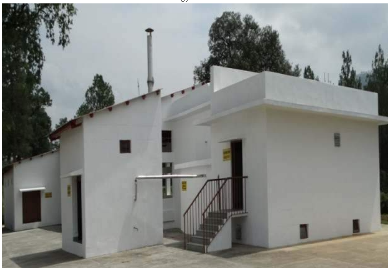
Fig 6.24. Compost pasteurization facility developed at VPKAS, Almora
